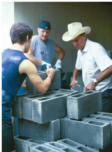
PIM team members playing jump rope with children (above) and moving concrete blocks (below).
