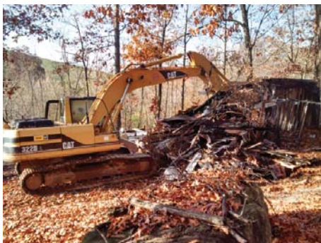
Partners Excavating demolishes the damaged structure. Photo: Jaime Miller Gonzalez
