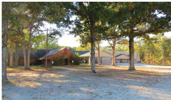
The Powhatan Mennonite Church building with the new addition dedicated over the celebration weekend.
