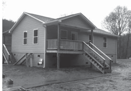
The completed house in Clendenin, W.Va. Photo: Clyde Kratz
